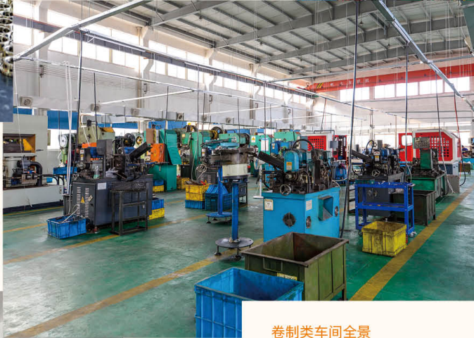
卷制类车间全景 Panoramic view of rolling workshop
